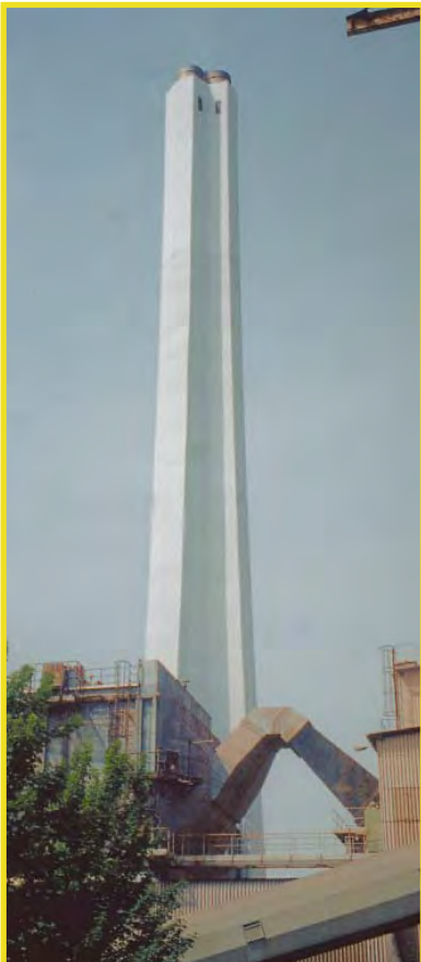
Left: Architectural masterpiece. This concrete structure houses three individual chimneys and its construction represented a major piece of investment for environmental protection. The emission situation around the plant was significantly improved, while its purposeful form represents quite an advertisement for the use of concrete in an industrial environment.
